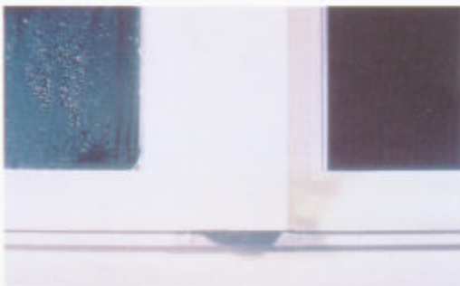
Left: Conventional IG; aluminum spacer; 2 lights of 3mm clear glass; 0.5" air space. Right: Improved IG; Intercept insulating glass spacer; Sungate 100 coated glass; argon gas fill.
